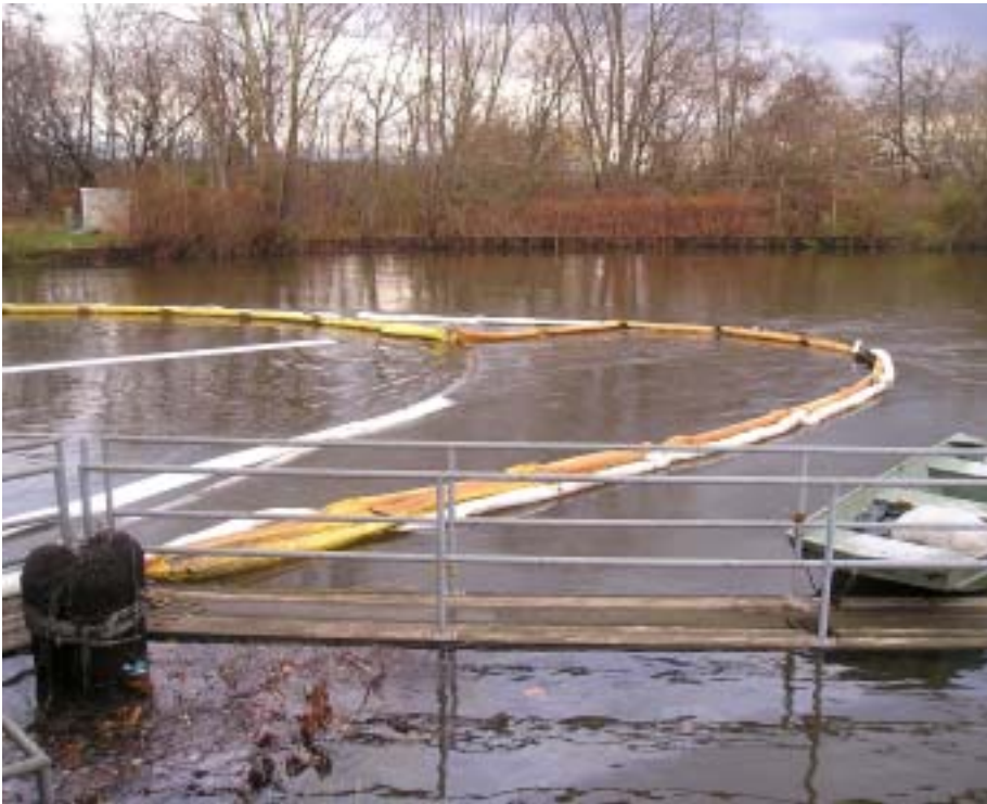
Absorbent and containment booms in place across Raccoon Creek, near the mouth.
