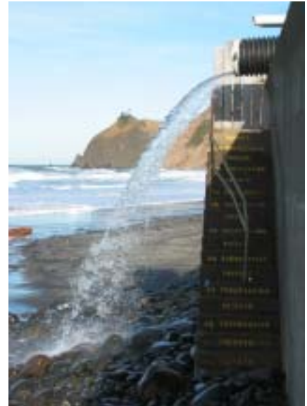
Storm drain outfall discharging to beach.
