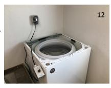
17. Carefully loop this cable to not strain or kink any of the wires. Secure with zip-ties back to the machine using the previous wiring harness tab.
