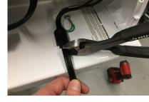
Cut off the tubing and wires from the control panel (they are not needed).
