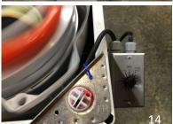
10. Attach the corner bracket to the electrical box through one of the knockout screw holes. (use a hammer to break the bump out) predrilling a small hole in the box may be needed and secure using selftapping screws.
