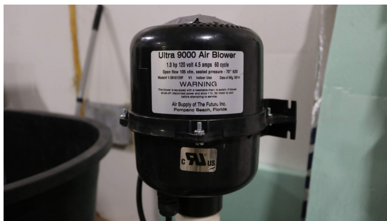
A common 1 hp jacuzzi blower from Air Supply of the Future, Inc. Consider mounting the blower away from the wash area to limit noise in the room and prevent water damage to blower. A dimmer switch and timer may also provide convenience.
