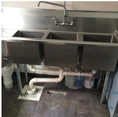
If your drain is underneath the sink then a twist drain makes it easy to drain the water without crawling underneath.
