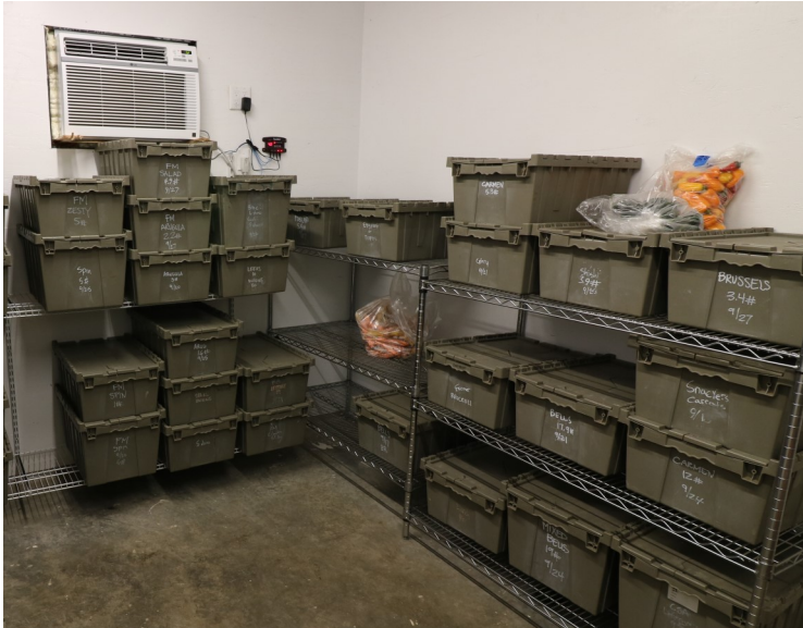
▲ The walk in cooler (10’x14’) is powered by a window AC unit and a CoolBot. It has a floor drain for easy clean out. Plywood painted walls, and wire racking to hold Buckhorn bins packed for deliveries.
