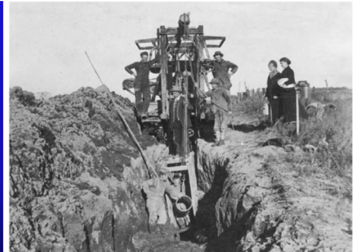
Laying subsurface drain tile with a machine. Shallow tiles and ditches were generally dug by hand. About four miles west of Dawson, Lac qui Parle County, circa 1905. (MHS photo)
