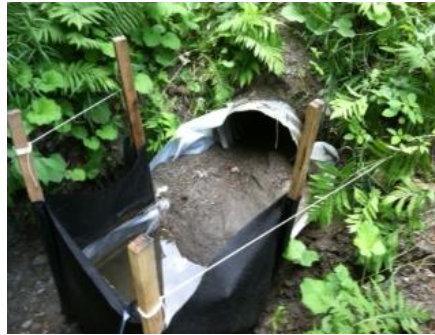
Figure 7: Silt fence constructed of plastic sheeting to retain sediment and filter fabric to pass stormwater, installed at culvert outlets to trap material eroded from roads and roadside ditches.
