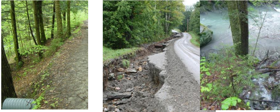
Figure 1: Evidence of water quality impacts associated with unpaved roads in Vermont's uplands: erosion of rills and gullies on impervious road surface (left panel), eroded roadside ditch resulting from channelized stormwater runoff (middle panel), direct discharge of road runoff to receiving stream from road culvert (right panel).
