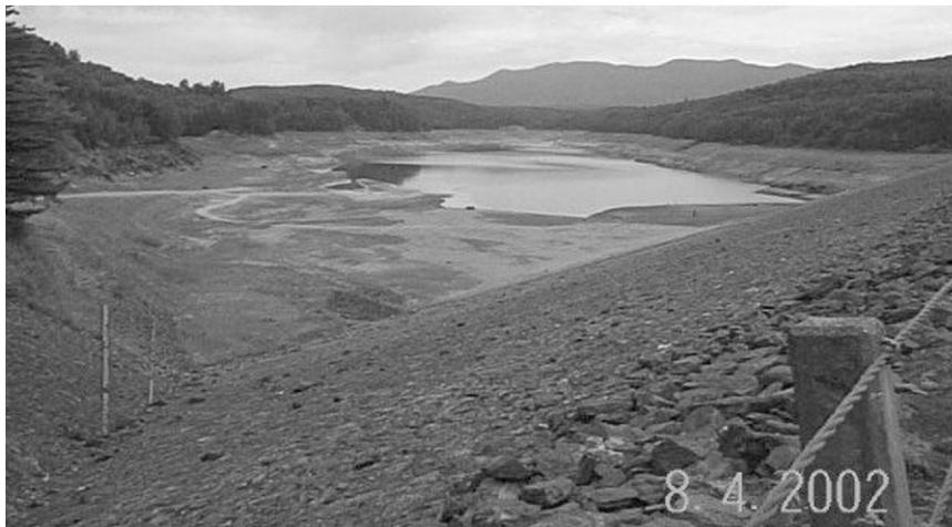
Figure 2. Waterbury Reservoir looking upstream from the dam during extreme drawdown for dam repair in early August 2002. Water level elevation shown is approximately 157.6 m, compared to a typical summer elevation of 179.8 m, shrinking the lake to <20% of its normal area.
