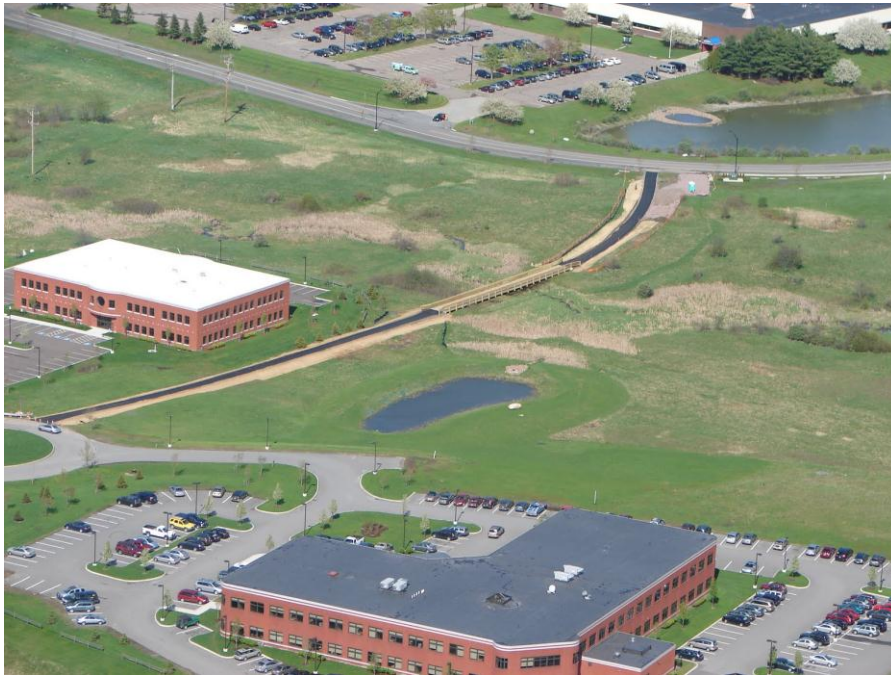
Figure 6: Aerial View of Tilley Drive Medical Facilities
