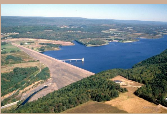
Figure 1. An Image of Beltzville Lake. Built by the US Army Corps of Engineers as a means of Flood Control for the Lehigh Valley.
