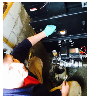
State Line Biofuels demonstrated a waste oil boiler to heat the biodiesel processor and enable methanol recovery. The waste oil boiler was selected due to the potential to use glycerin, a co-product of the biodiesel process, as a fuel source.
