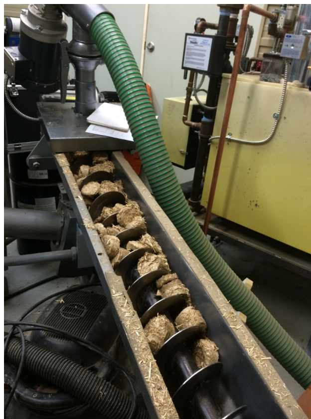
Grass pucks being fed into an EvoWorld HC100 Eco boiler at Meach Cove Trust in Shelburne, VT.
