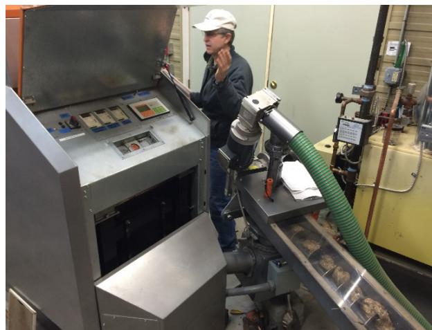
Chris Davis explains the details of the EvoWorld HC100 Eco to visitors at Meach Cove Trust. The boiler was designed in Austria, but is made in the US under a license by Troy Boiler Works (Troy, New York). It was intended for wood chips, but has been successful at running on grass pucks.
