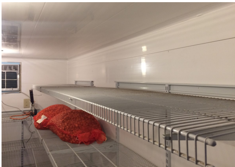
Smooth, clean and shiny, this CoolBot™ cooler used TrussCore™ twinwall PVC as a finish surface.
