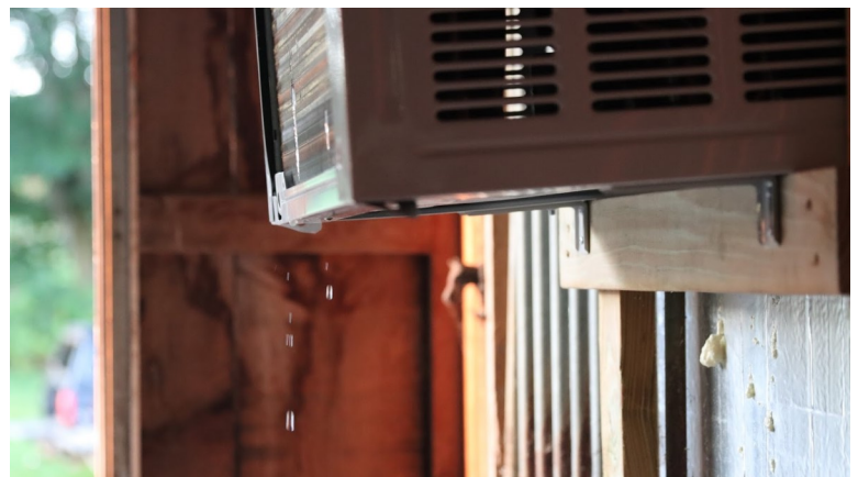
The AC unit should be installed with a slight pitch out and down to ensure water flows away from the wall and produce.
