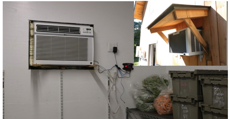
CoolBots need to be kept clean of leaves, dirt and debris, this farm installed a small roof to keep their investment protected, and properly sloped the unit to drain outside the building.
