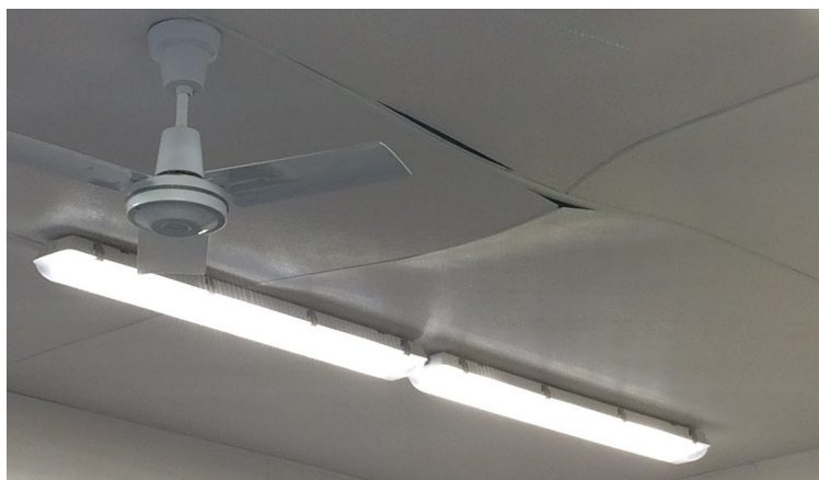
FRP or dairyboard is a common, washable finish surface in coolers and wash/pack areas. Pay close attention to appropriate adhesives and follow the installation instructions to prevent delamination.
