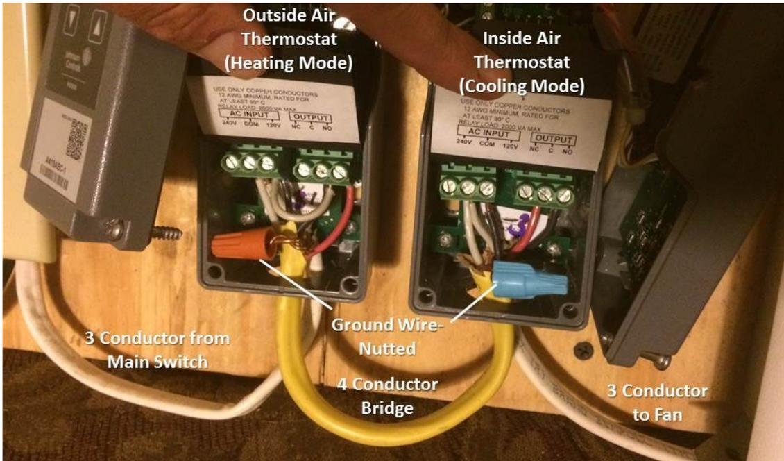
This shows the actual wiring of the thermostats (Johnson Control A419's in this case.) Note the use of 4 conductor wire between the two thermostats to allow both full-time power to the second thermostat's display and switched power to the controlled terminals.
