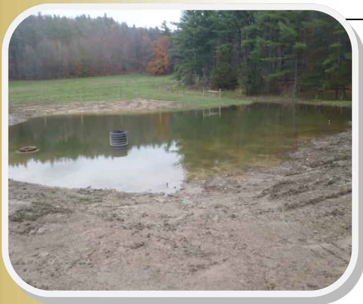
Rehabilitated farm pond with overflow and water intake structure installed. Fence was built to exclude livestock from pond and stream.
